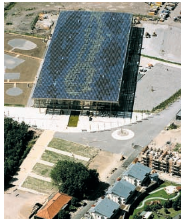
Figure 195 Academy Mont-Cenis Herne-Sodingen, Germany
