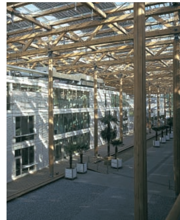
Figure 196 Interior showing primary structure
