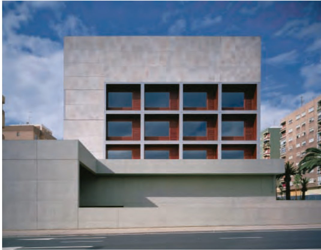
8, 9. The museum asserts itself against the busy street. 10. A prominent staircase connects the exhibition areas.
