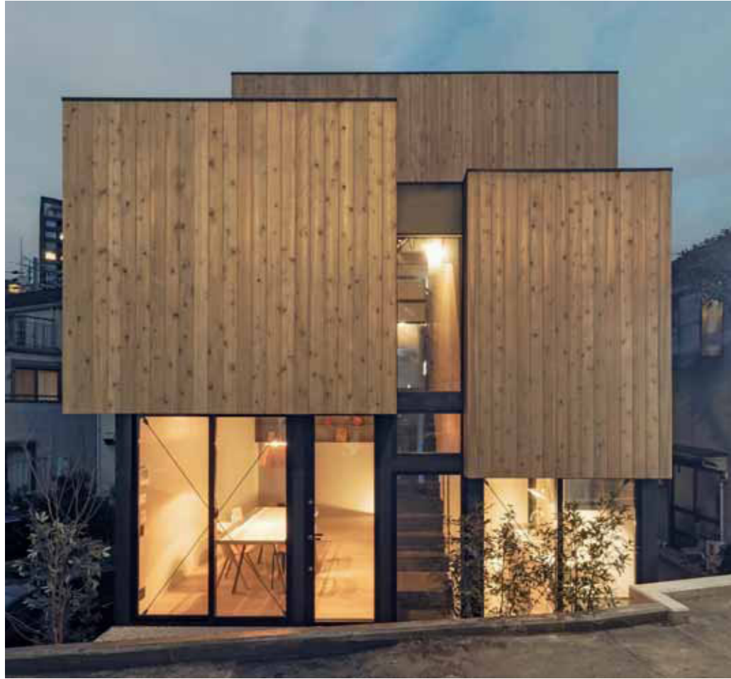
The In-between House in Tokyo, Japan, by YUUA is an example for insertion of small sized home into a densely built area.
