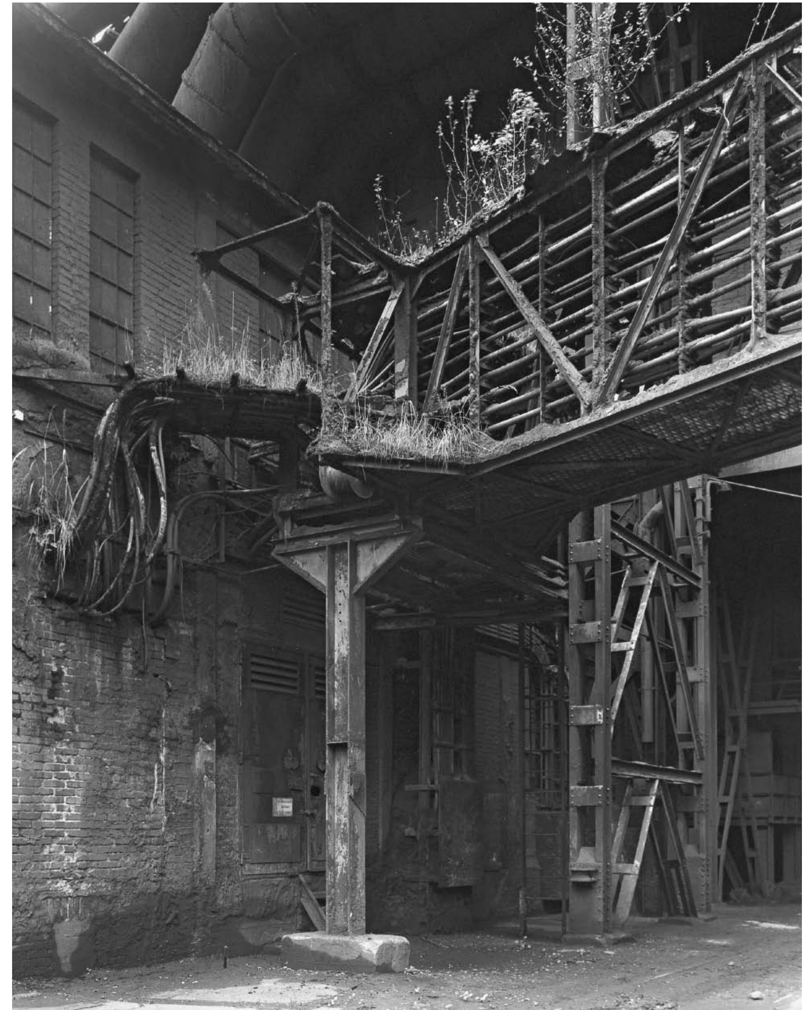
8, 9. The various ore-dressing processes are accommodated in the tightest possible space. A complicated system of conveyor belts, pipes and bridges provides the necessary links.
