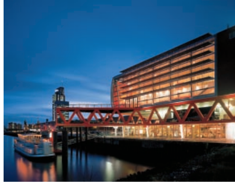
South Elevation; sun louvers and delivery-ramp lean out over the Rijnhaven quay. The taxi-boat pontoon (by Drost and van Veen) delivers direct to the terrace of the »Leipzig« restaurant. By night – the concept of free ground plane, sandwiched service and suspended foyer – the robust language of harbours – a formal and functional clarity.
