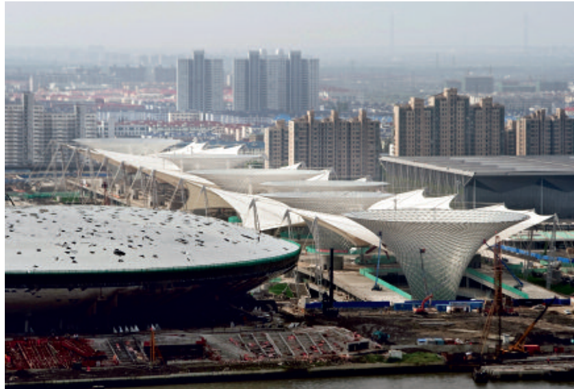
Fig. 13 Megastructure - Expo Shanghai 2010, Knippers Helbig Advanced Engineering
