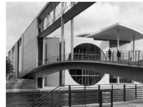
Façade facing the Spree River
